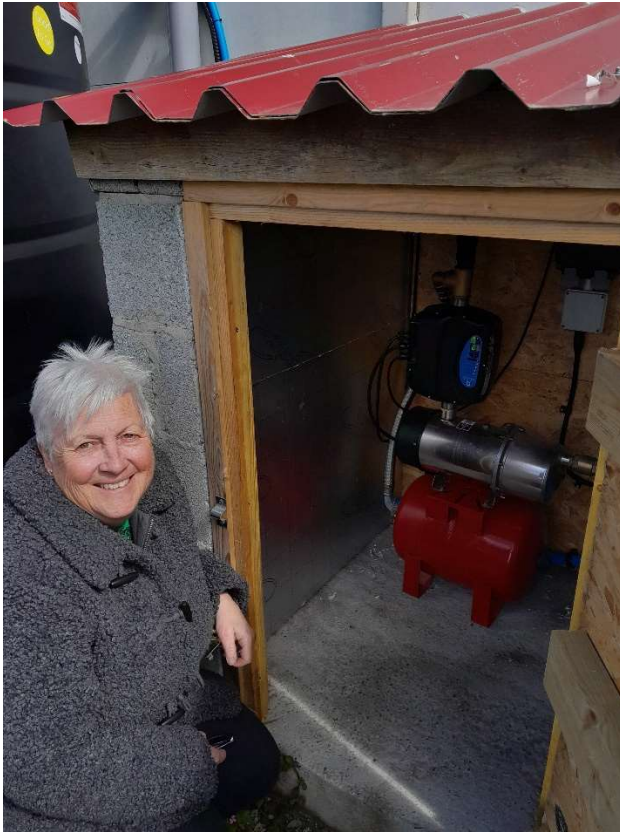
Sian James and the pump supplying rainwater to toilets and washing machines
