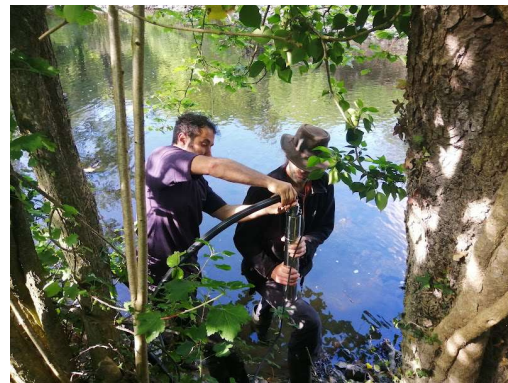
Installation of the pump in the river Summer 2022
