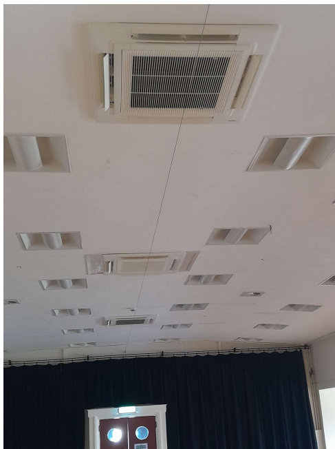
Heating air inlets in the main hall and in the kitchen. The main hall also has low energy lighting strips in the ceiling, also funded as part of the grant.
